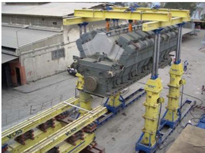
Mounting of a diesel engine 280 tons at the powerplant in Chekka, Libanon
