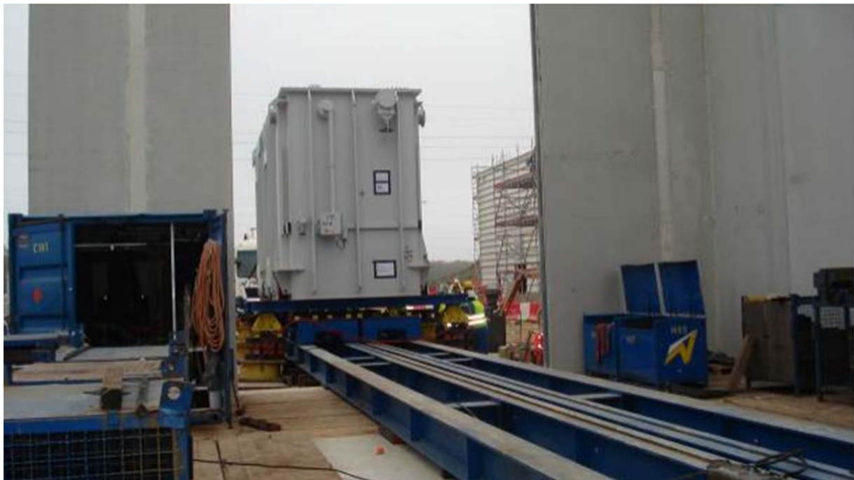
Moving a transformer with 210 tons over a pit onto the foundation
