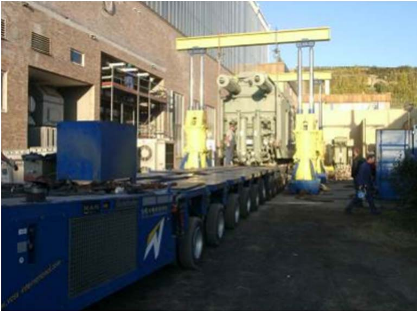
Unloading a transformer with 220 tons
