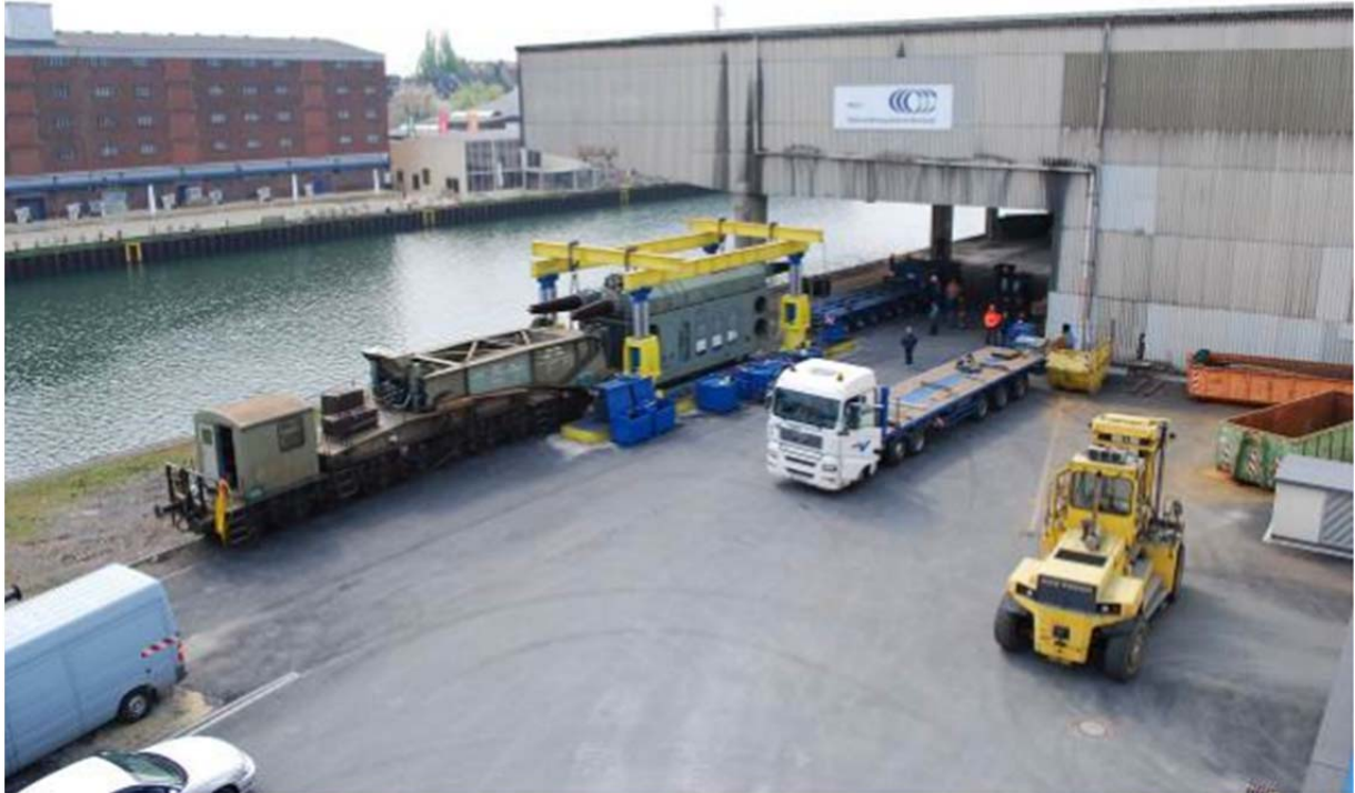
Unloading a transformer with 180 tons out of a railway wagon
