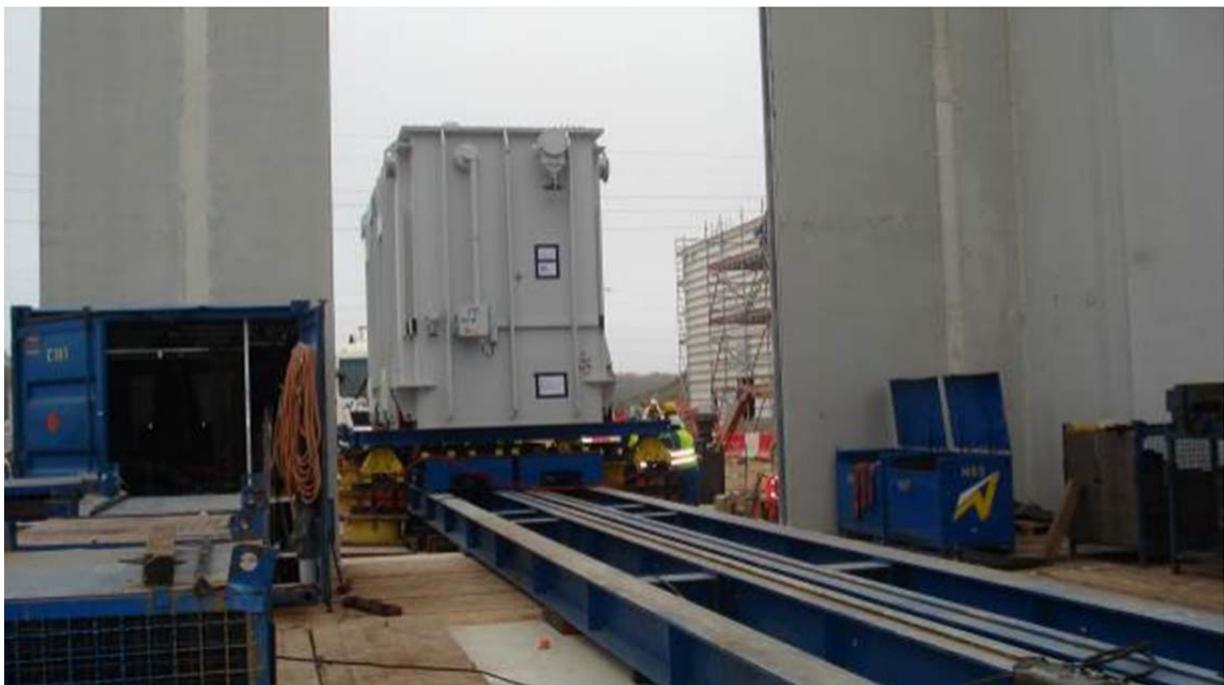
Moving a transformer with 210 tons over a pit onto the foundation
